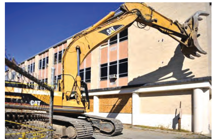
An excavator prepares to demolish portions of the former Vocational School.
