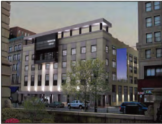
Renovated Telegram and Gazette Building for Quinsigamond Community College
