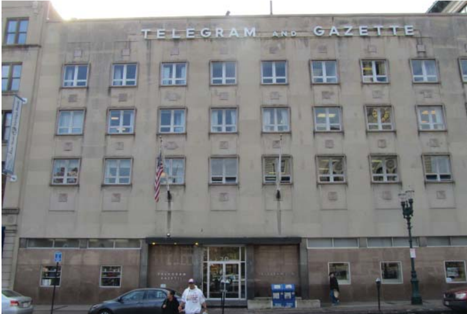
20 Franklin Street: existing Franklin Street façade.
