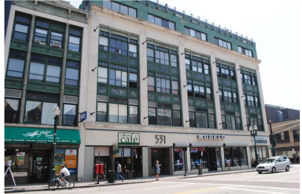
Former Filene's Building on Main Street.
