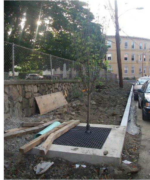
Stormwater tree pit under construction.
