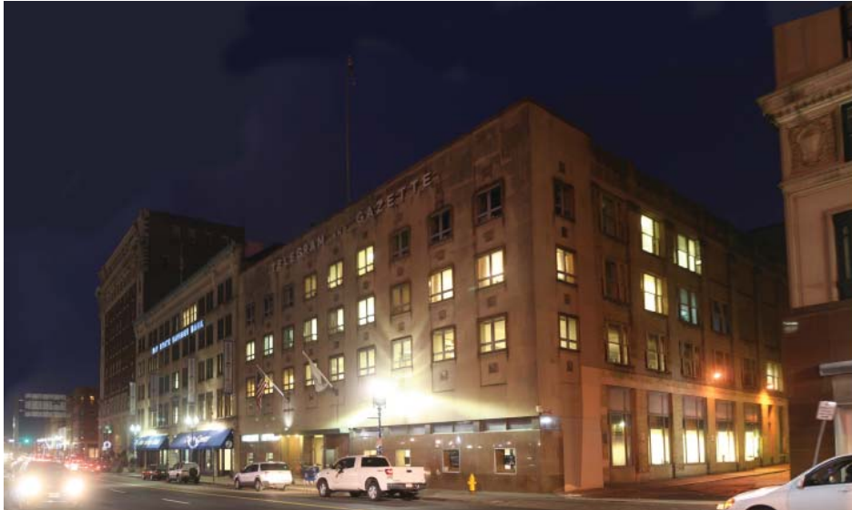
20 Franklin Street, Franklin Street façade, existing conditions.
