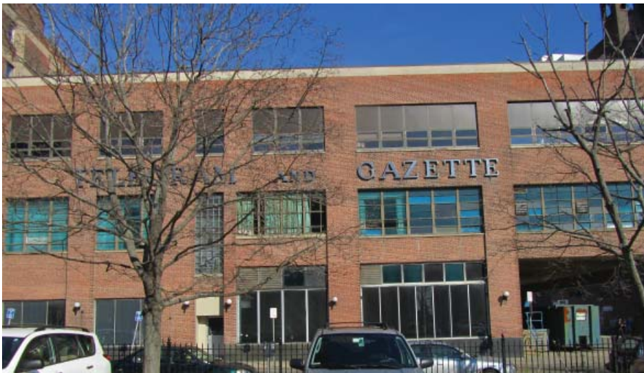
20 Franklin Street: existing Federal Street façade.
