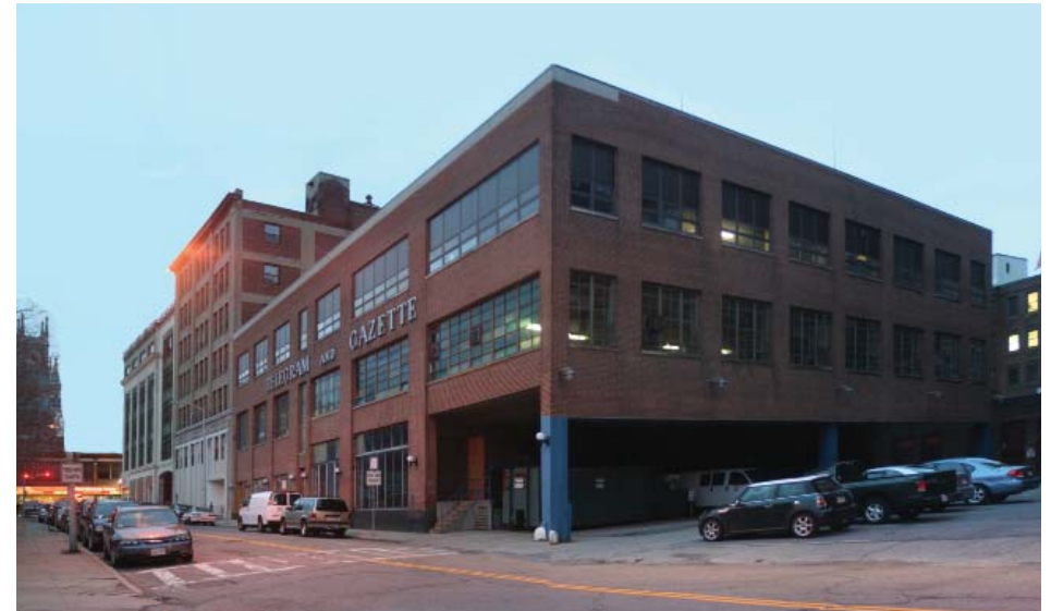
20 Federal Street, Federal Street façade, existing conditions.
